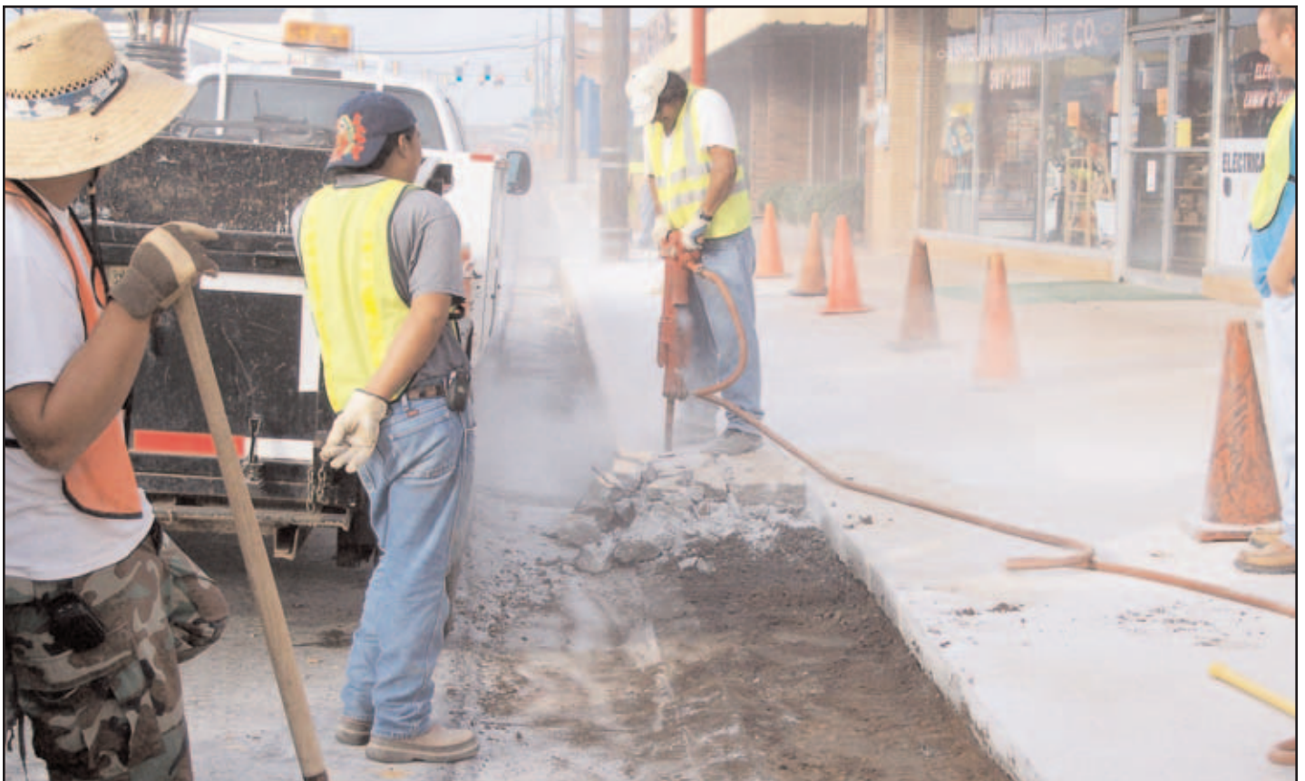
If you've ever scraped the front end of your vehicle on the second block of E. Washington, you'll be glad to know a new curb is in place there. The new curb should prevent the "bumper scrape" so common there for years. Photo Linda Sellars
